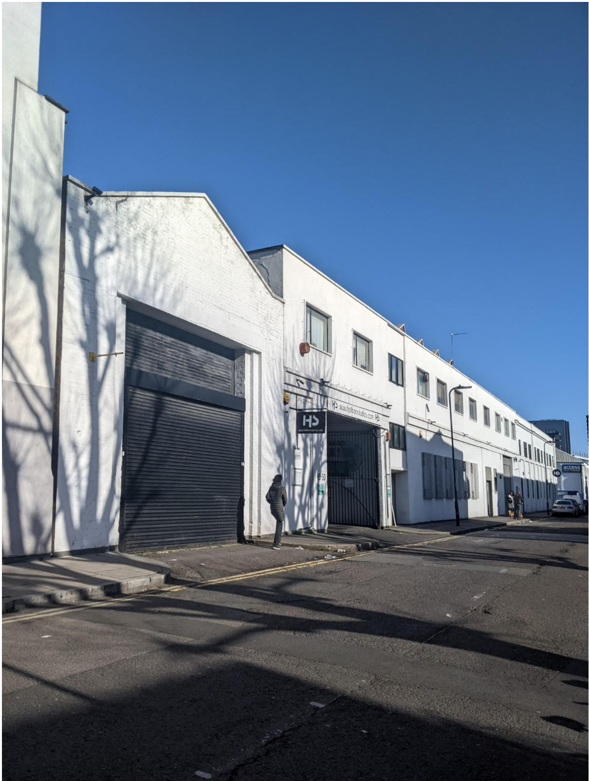
View from Eagle Wharf Road
